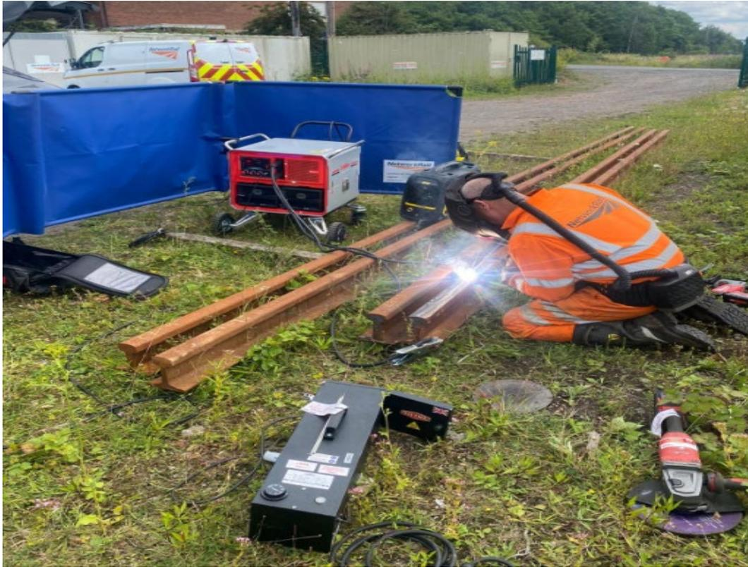
THIS BATTERY POWERED WELDING MACHINE IS BEING USED ALONG WITH ARC SENSING MIG/ MAG WIRE FEEDER IN EUROPE FOR RAILWAY TRACK MAINTENANCE
